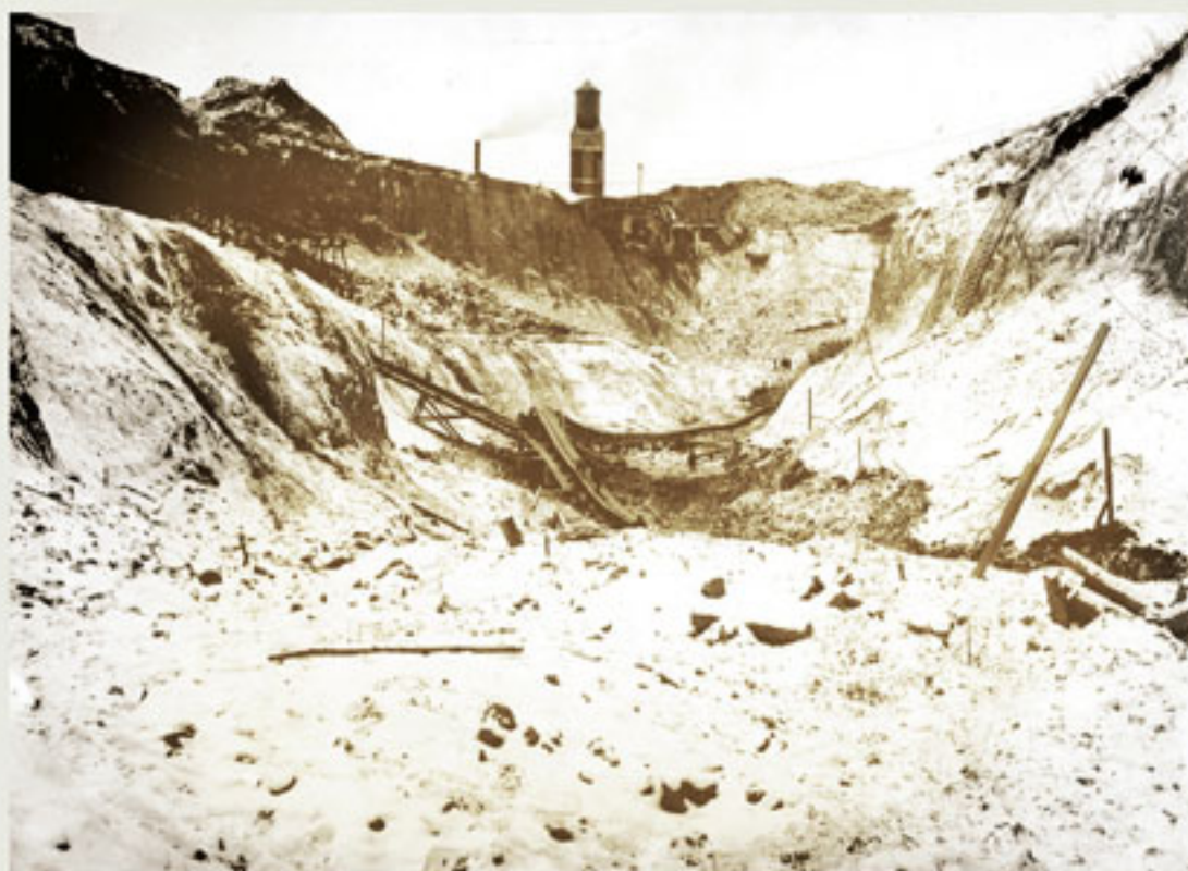
Quelques semaines après la catastrophe, les dommages sont impressionnants, aux abords de l'usine. On y remarque des installations ferroviaires en piteux état. A few weeks after the catastrophe, damages were impressive around the plant. One may see that the railway installations were in a very sorry condition. Source : Centre d'histoire Sir William Price / Centre d'histoire Sir William Price, CCHSWP C21//13
