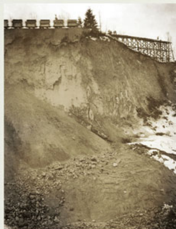
Au lendemain de la tragédie, on élabore des installations permettant d'acheminer le matériel de remplissage aux abords du gouffre. On the days following the tragedy, installations intended for carrying filling materials to the brinks of the abyss were put in place. Source : Centre d'histoire Sir William Price / Centre d'histoire Sir William Price, CCHSWP C21//25
