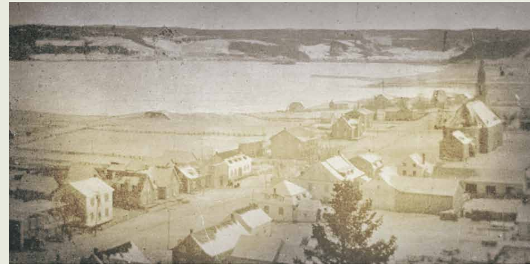
Rue Victoria, Bagotville/Victoria Street, Bagotville SHS-P2-S7-P00852-3
