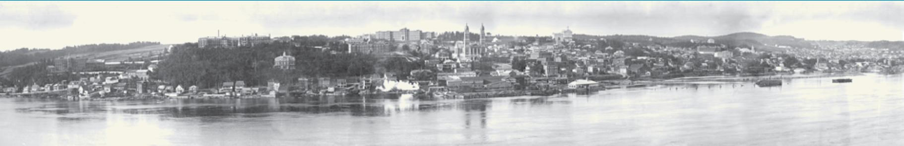
Vue de Chicoutimi vers 1929 (le port est en construction) (BAnQ, Collection SHS, P2, S7,P13909) View of Chicoutimi around 1929 (the port is under construction) (BAnQ, Collection SHS, P2, S7,P13909)
